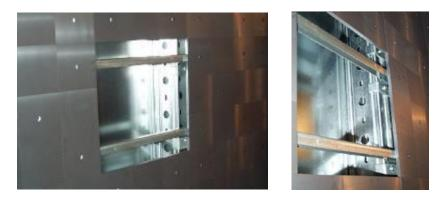
Ferrite panels are screwed onto a metallic sub-structure, made of main and secondary steel profiles. Vertical main profiles are directly fixed onto the shielded room, using the joining OMEGA profiles between two shielding panels. Then horizontal secondary profiles are screwed onto these main profiles.
